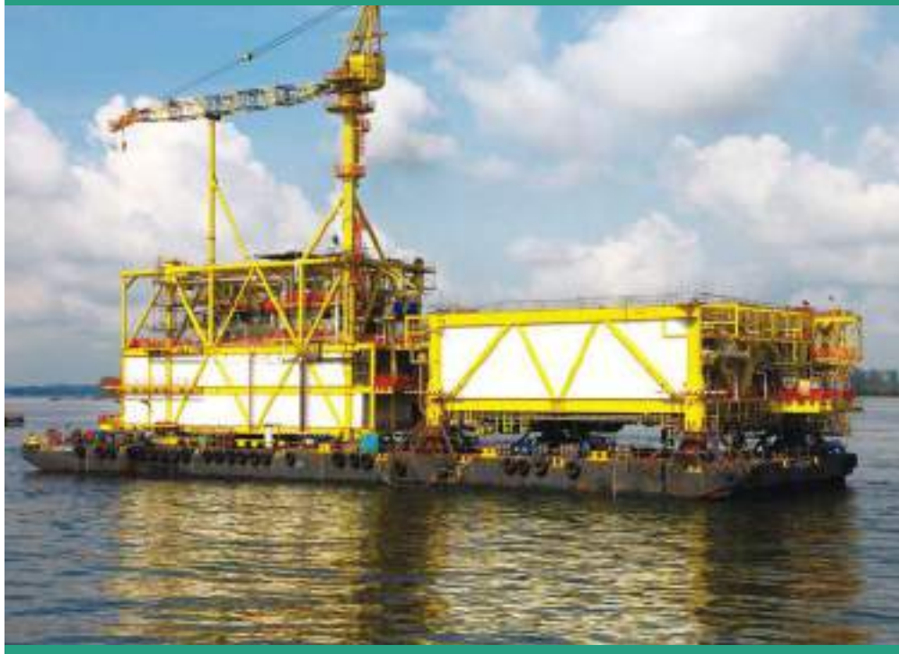
The load out of Kinabalu non-associated gas topside
