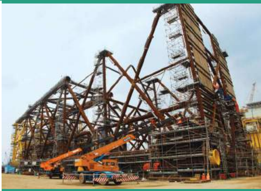
F14 topside under construction in MMHE West, Pasir Gudang
